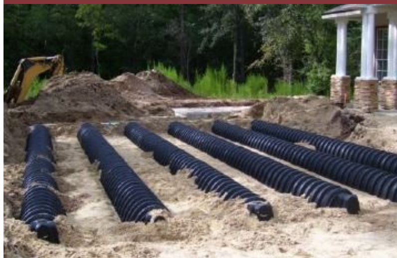
Septic drain field pipes
